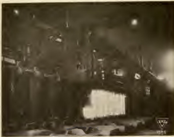
STRIPPING MOLDS FROM THE INGOTS
